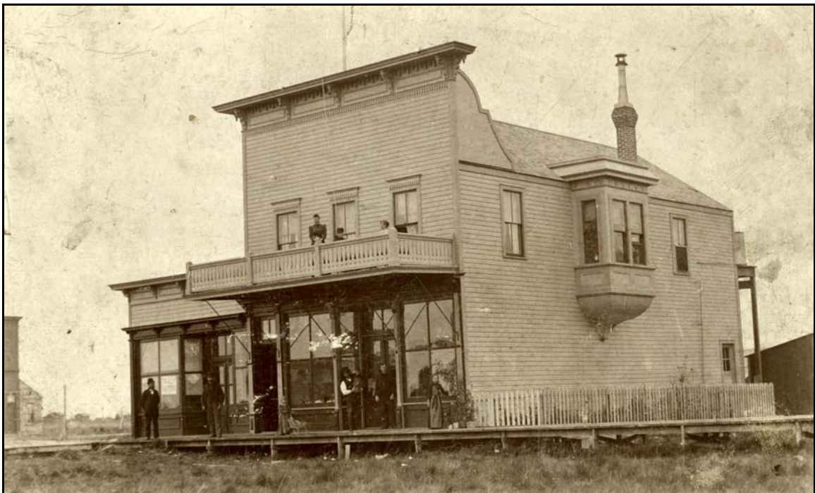
Figure 29: High false front parapet disguises the simpler structure behind this Ocosta Store, 1890-1920, Polson Museum Collection.
