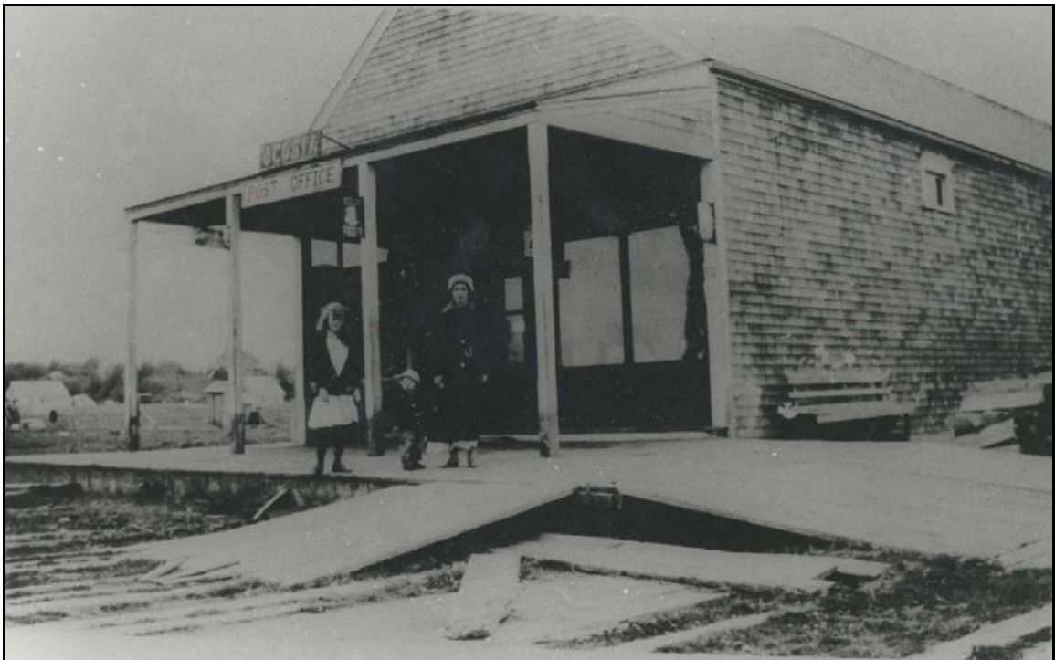
Figure 39: Ocosta Post Office, 1890-1908, Aberdeen Museum Collection.
