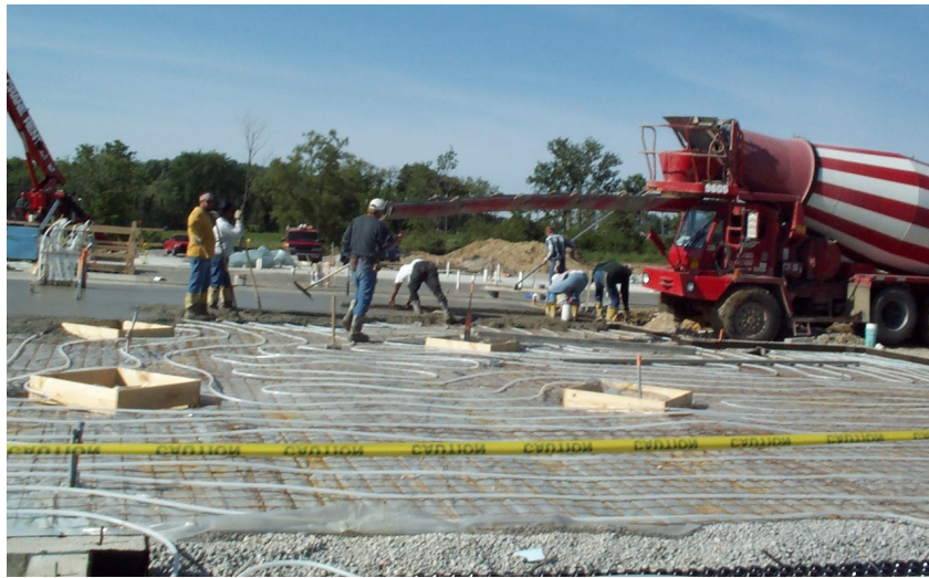
Figure 14: Hydronic Radiant Floor Heating System Installation
