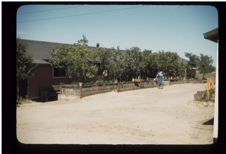
Figure 41: Amache Barracks, Courtesy of the Amache Preservation Society, the McClelland Collection.
