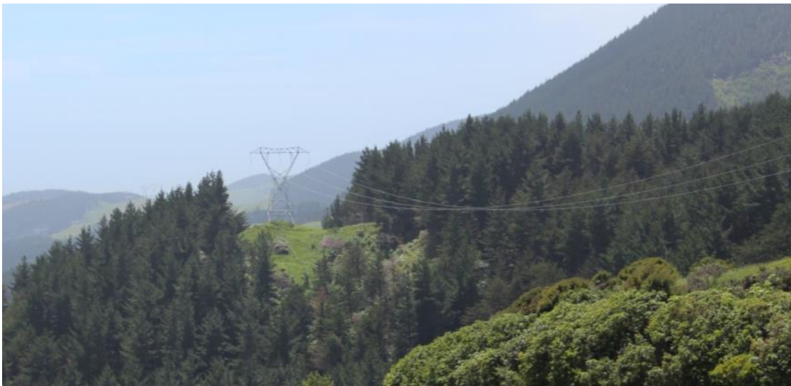
Figure 4: Transmission line structure in New Zealand. The salt laden ocean winds cause large problems with corrosion.
