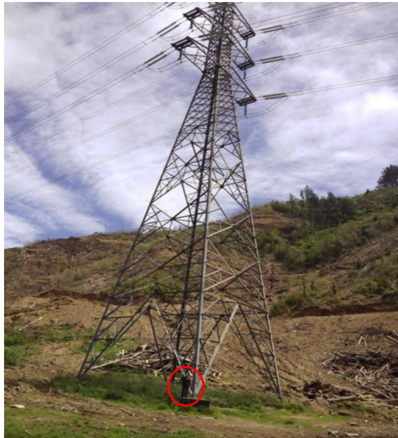
Figure 6: The author standing on the foundation (circled) shows the scale of a typical transmission line tower located in New Zealand.
