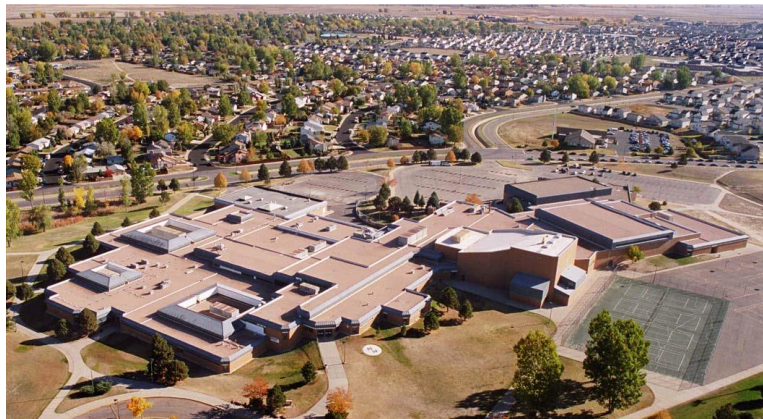
Figure 3. Aerial photograph of the former Montbello High School building and surrounding Montbello Neighborhood (source: http://danddroofing.com/portfolio/montbello-high-school/ ).
