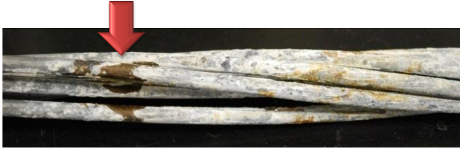
Figure 44: The loading bearing steel core in ACSR after being partially submerged in 85 o C, 3 wt. % seasalt for 104 days. The red arrow shows spots where the galvanization is lost.
