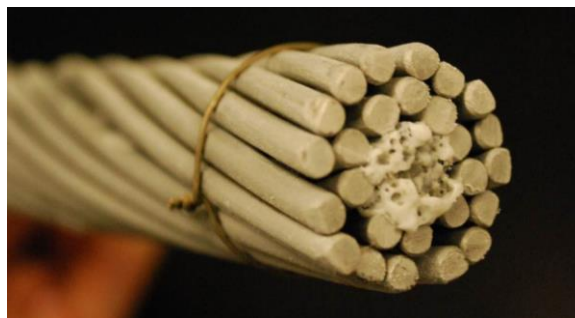
Figure 68: Build-up of corrosion products at the end of the ACCR core. Picture taken on day 7 of 104 in Test A.
