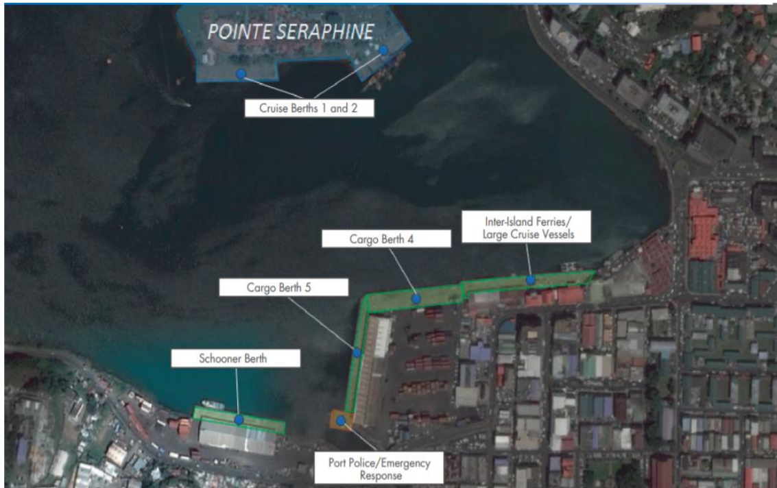
Figure 9: Aerial View of Port Castries (SLASPA 2016)
