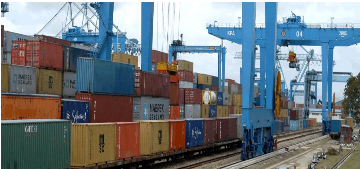
Figure 11: RMG Cranes at Berth 16, Terminal I-Mombasa Port. Source KPA
