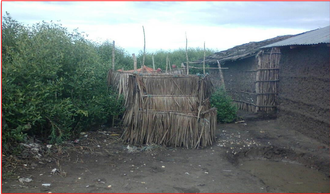
Figure 36. Precarious Toilet used for Shower only at Icidua
