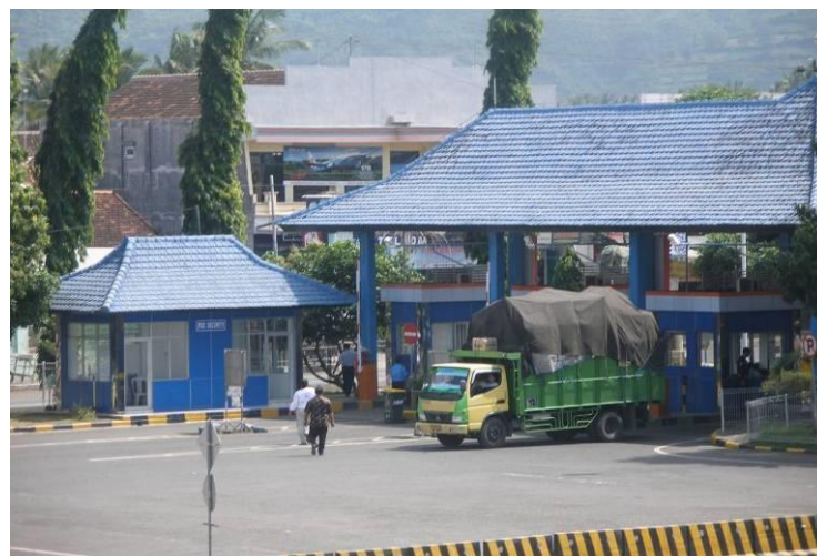
Figure 4-5. Ticket counter on the gate of vehicle path
