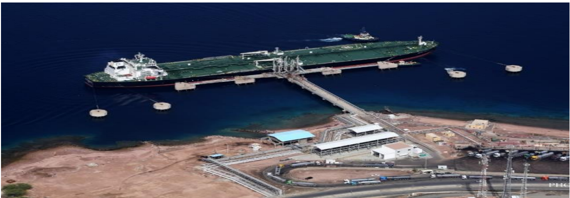
Figure 12: Oil Terminal Source:( ADC, 2015)
