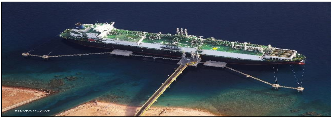
Figure 11: LNG Terminal Source: (ADC, 2015)
