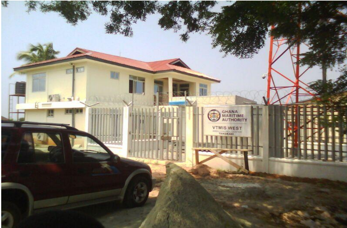
B: VTMIS West Control Centre (WCC)
