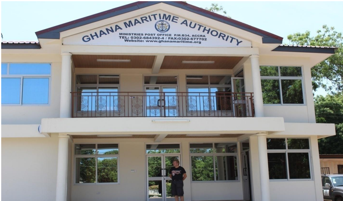
A: National Control Centre at GMA HQ
