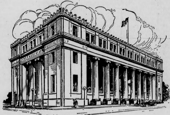
Home Office Building Fourth and Broadway
