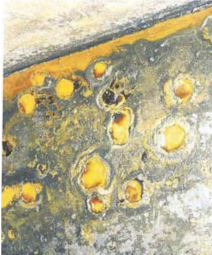
Fig. 20. Bacterial corrosion (Source: DNV paper series No.2000-P008. p.15)
