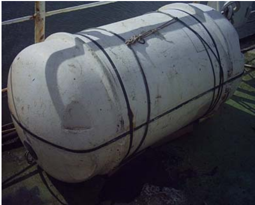
HRU and markings missing.
