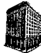
Provident Bank Building
