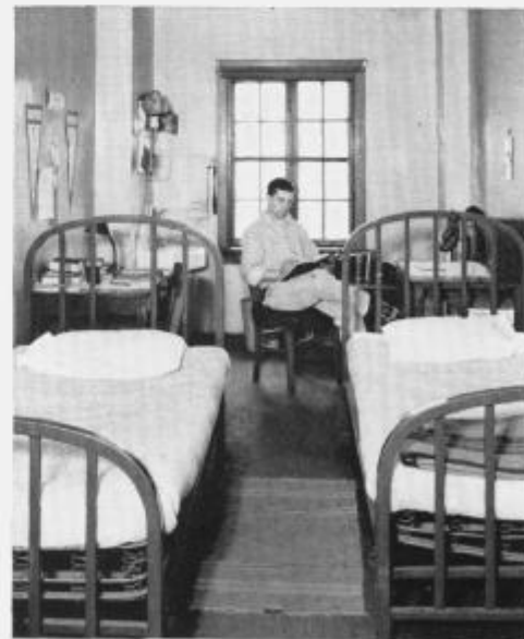
Typical room scene in Elet Hall.
