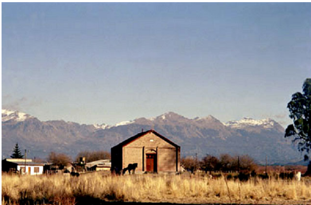
Figure 4. The disused Bethel Chapel, Trevelin.
