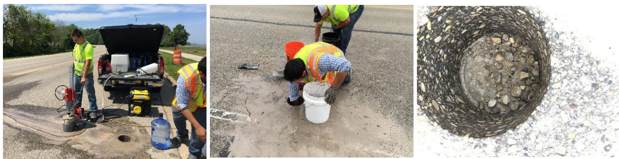
(a) WisDOT coring rig at STH 32
