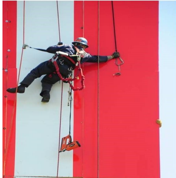
Figure 4: CG employee working on hanging a day board on a navigational aid. Photo courtesy of ET1 R. Beatty, USCG
