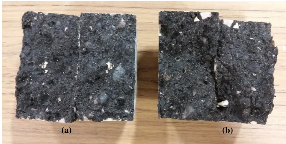
Figure 5.7 Representative Sample Exposed to (a) Dry Condition (b) Moisture Damage
