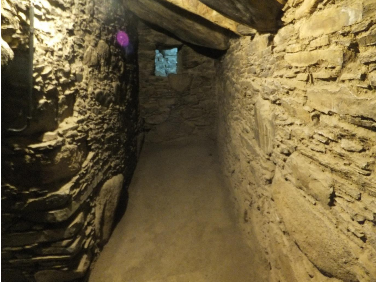
Figure 2.13. Image inside third floor of Chullpa in Willcawain. Note the slanted roof.
