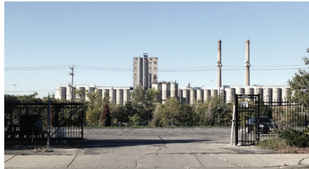
view of site from W. Pierce Street
