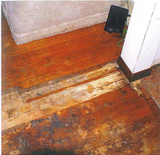
Lighter floor boards show where a wall once stood.
