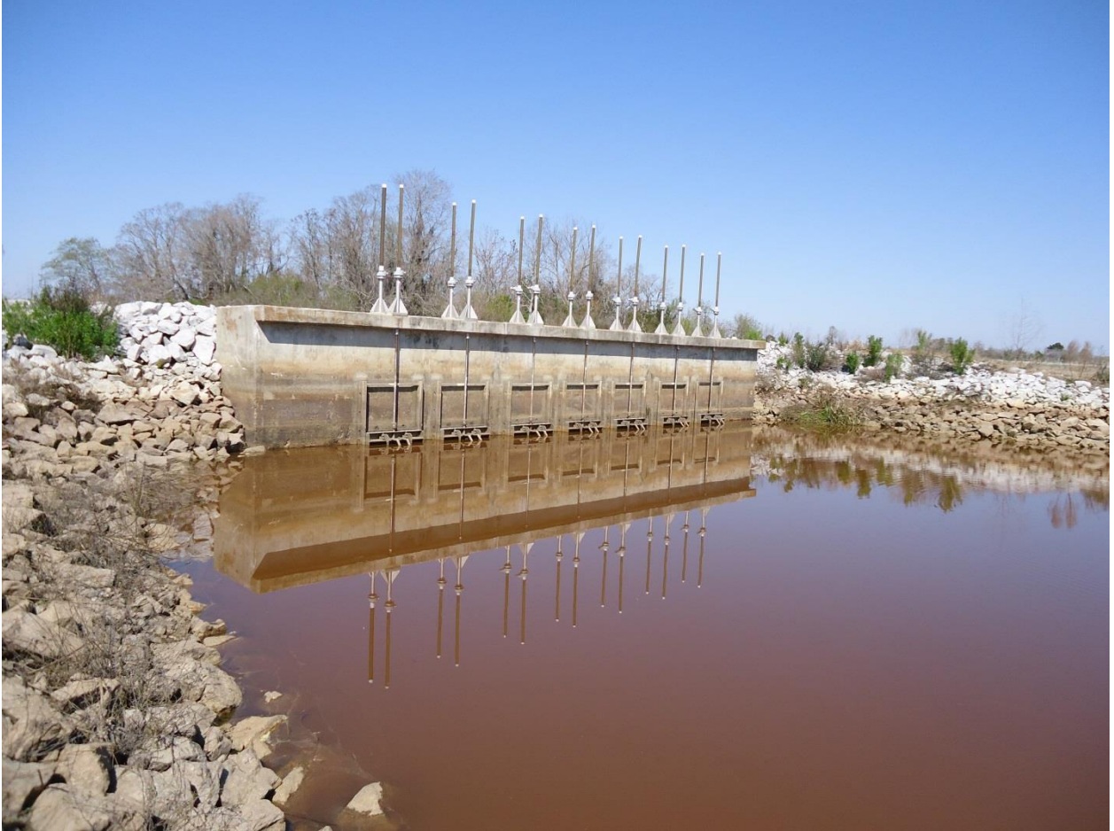
(Figure 9. The freshwater supply canal and water control structures. Photo: author. )
