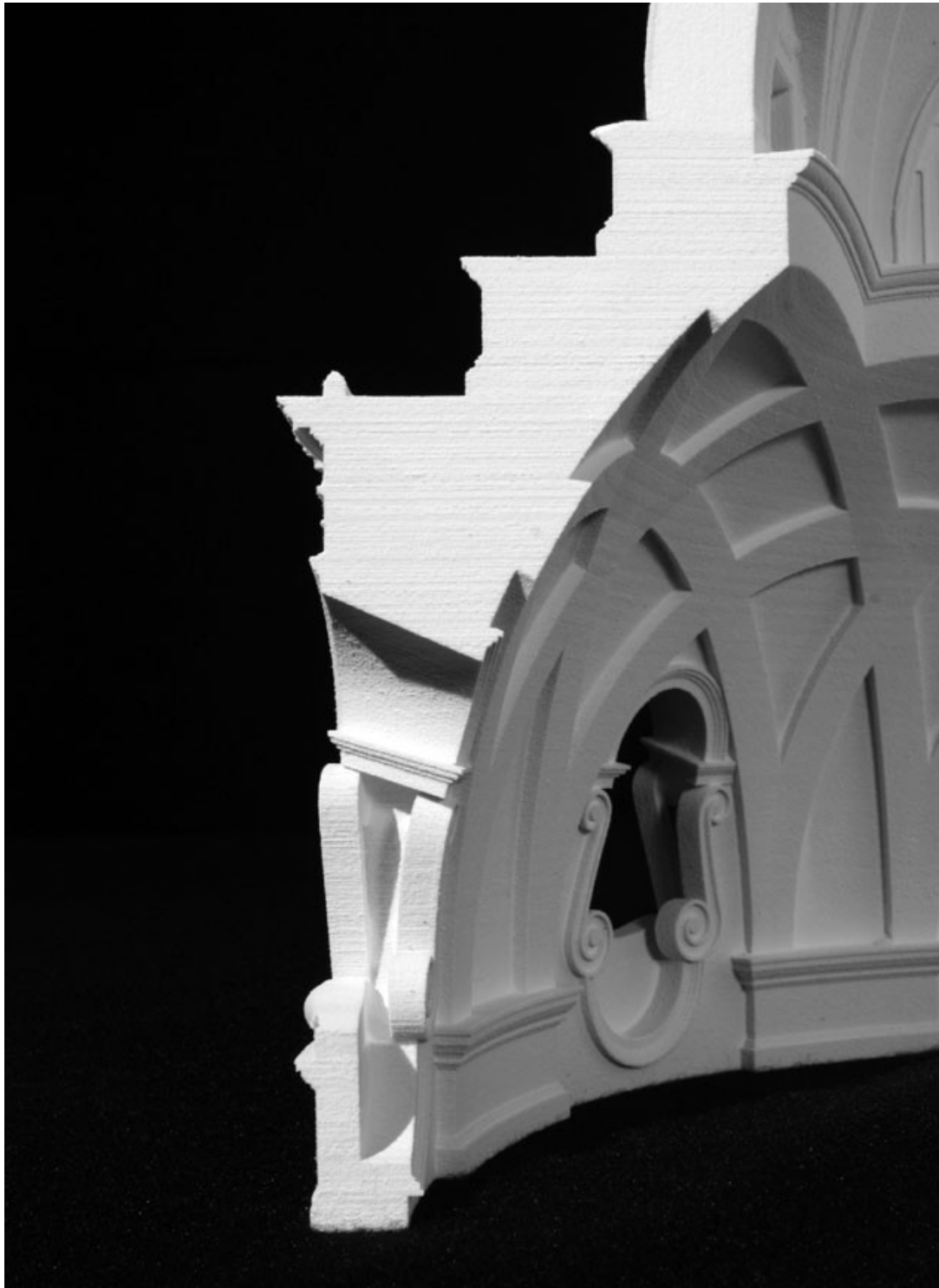
Figure 183. Section detail of the gallery windows. Picture of the 3d printed model by the author.
