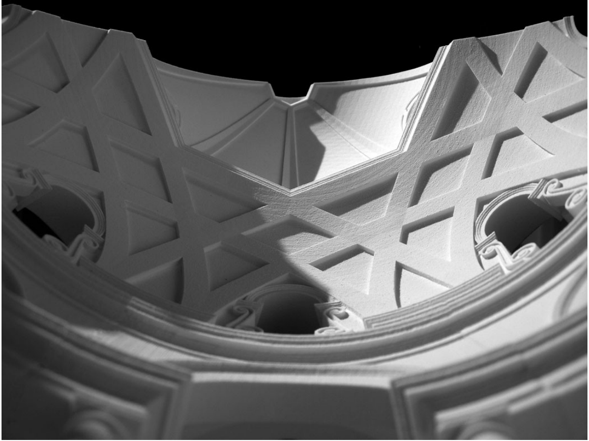
Figure 166. View of the interlaced ribbed dome. Picture by the 3d printed model by the author.
