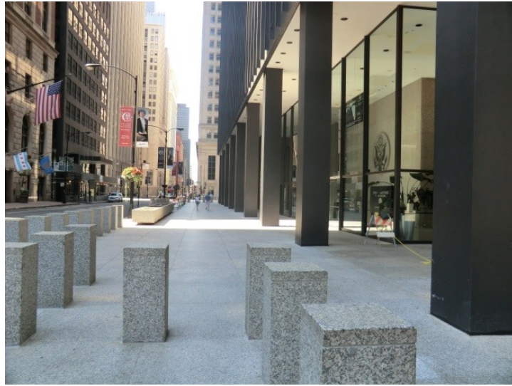
Figure 10: Bollards surrounding Dirksen and Kluczynski federal buildings
