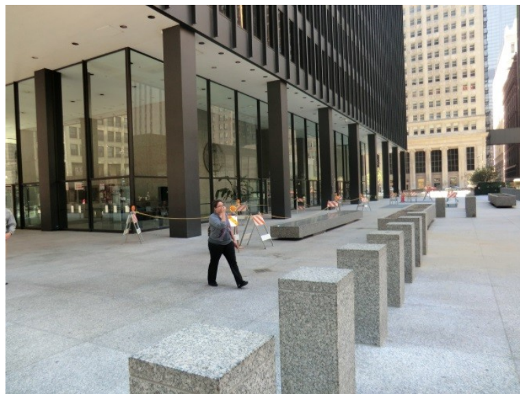
Figure 11: Bollards and planters surrounding Dirksen and Kluczynski federal buildings
