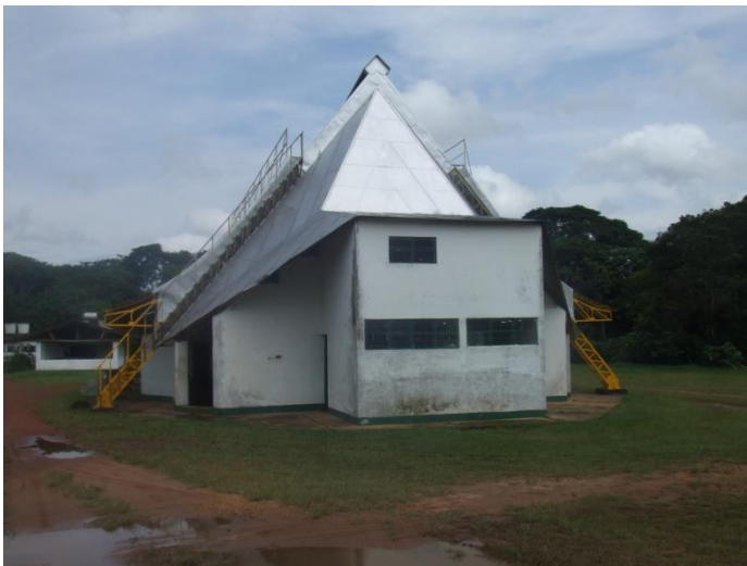
Figure 25: Las Gaviotas: Hospital. Source: Author's Photo.
