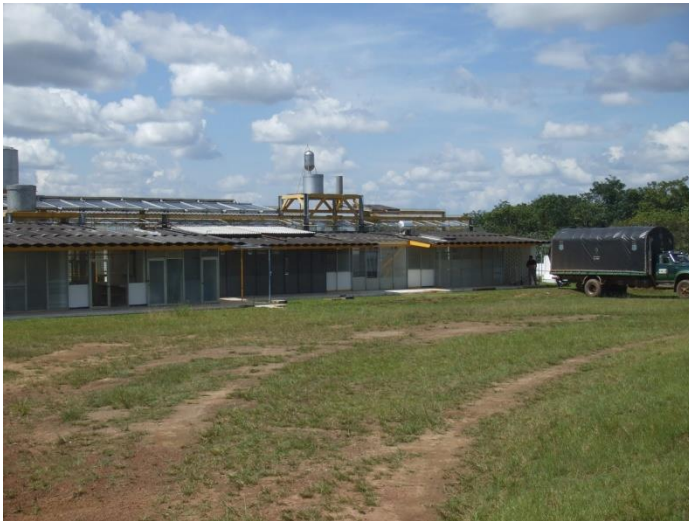
Figure 27: Las Gaviotas: Water Purification Plant. Source: Author's Photo.
