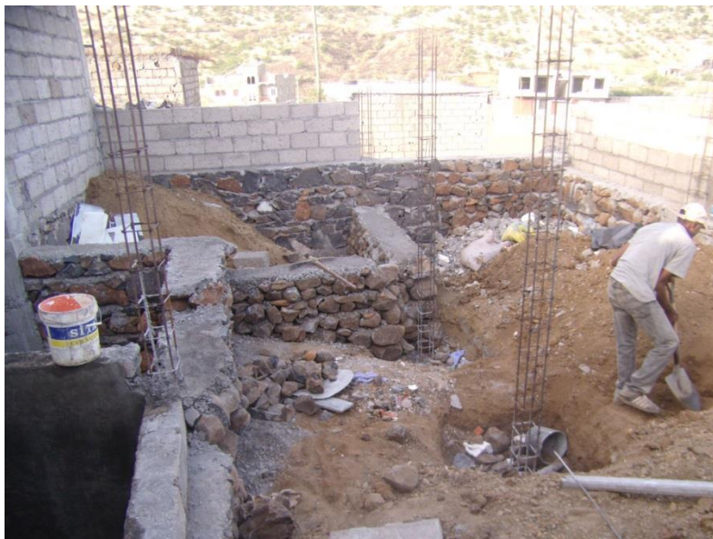
Figure 49: Foundation Construction Source: Learner's photo
