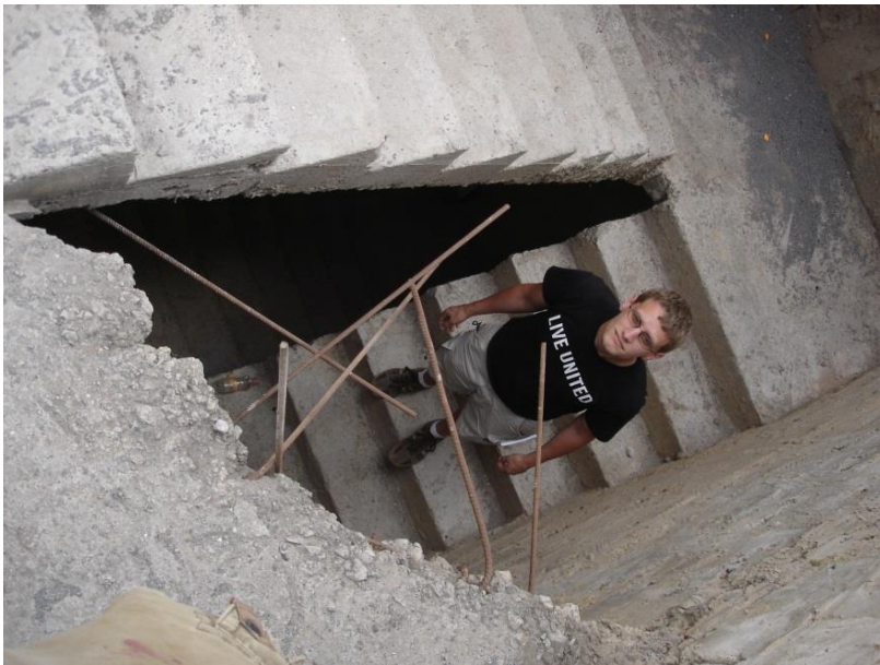
Figure 9: Learner Observes Unfinished Construction. Source: Learner's photo.
