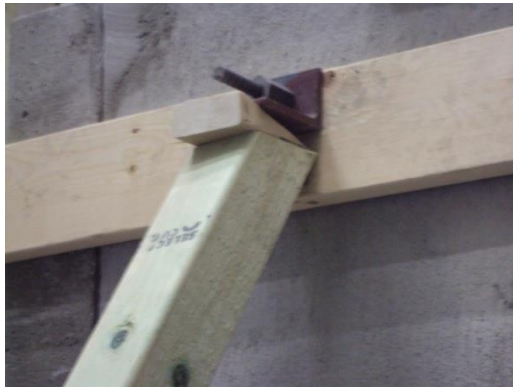
Figure 4.14: Panels installation; (a)Lifting a panel, (b)Installation of panels, (c)Temporary lateral Supports, (d)Detail of lateral supports at top (left picture) and bottom (right picture).
