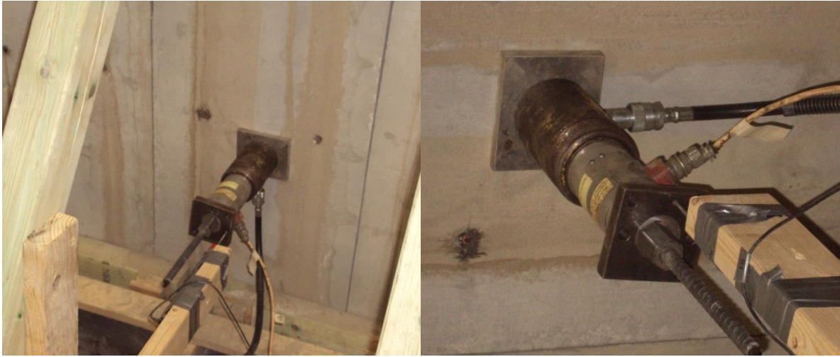
Figure 3.32: Pullout test on CLSM abutment at wing walls.
