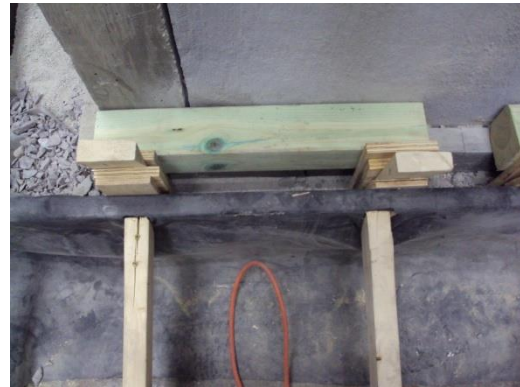
Figure 4.14: Panels installation; (a)Lifting a panel, (b)Installation of panels, (c)Temporary lateral Supports, (d)Detail of lateral supports at top (left picture) and bottom (right picture).
