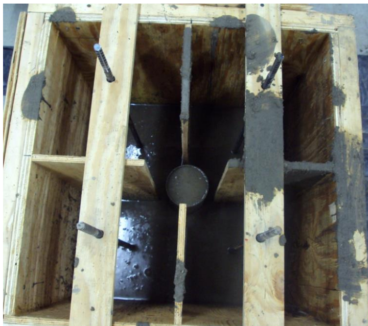
Figure 3.27: Cylindrical molds placed in the center of the box.
