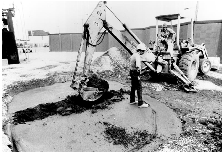
Figure 2.2: Excavating CLSM with backhoe (ACI 229R, 1999).
