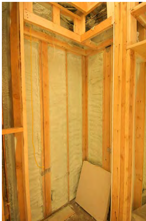
Figure 1.20 Insulation is used to limit the conduction of heat from the inside to the outside (in winter) and from the outside to the inside (in summer). (credit: Giles Douglas)
