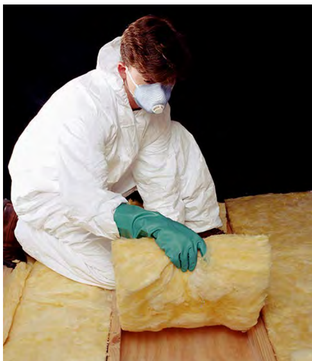
Figure 1.23 The fiberglass batt is used for insulation of walls and ceilings to prevent heat transfer between the inside of the building and the outside environment. (credit: Tracey Nicholls)
