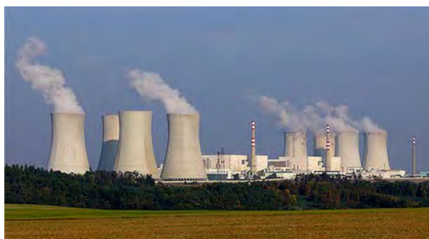
Figure 4.5 The heat exhausted from a nuclear power plant goes to the cooling towers, where it is released into the atmosphere.
