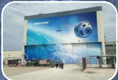
Comm. Crew & Cargo Processing Facility $20M
