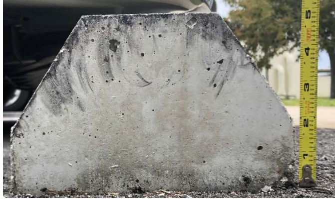
Figure 27: Parking Calk Height Measurement
