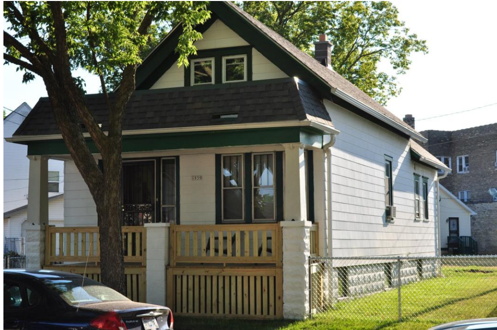
Figure 3-2 Existing Workers Cottage in Study Area (Source: Author)
