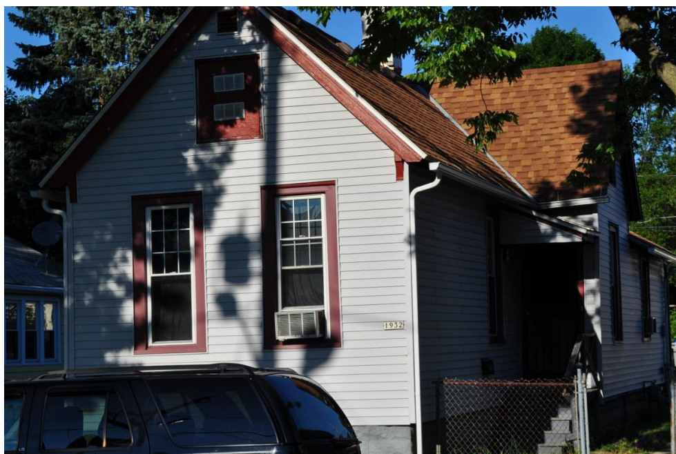
Figure 5-7: Existing Worker's Cottage from Group C that Underwent Rehabilitation Source: Author
