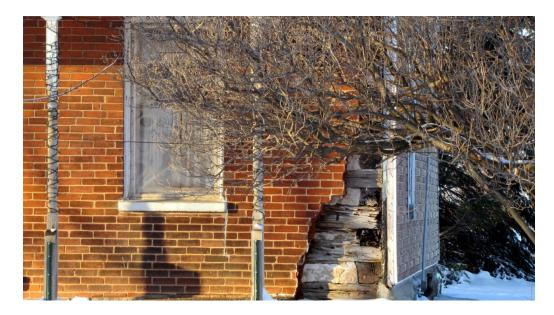
Figure 35: The log underneath a brick veneer on the Hayes home
