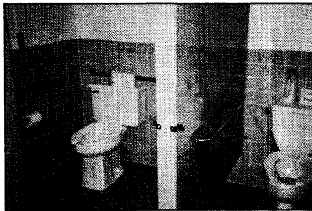
Men's toilet room.
