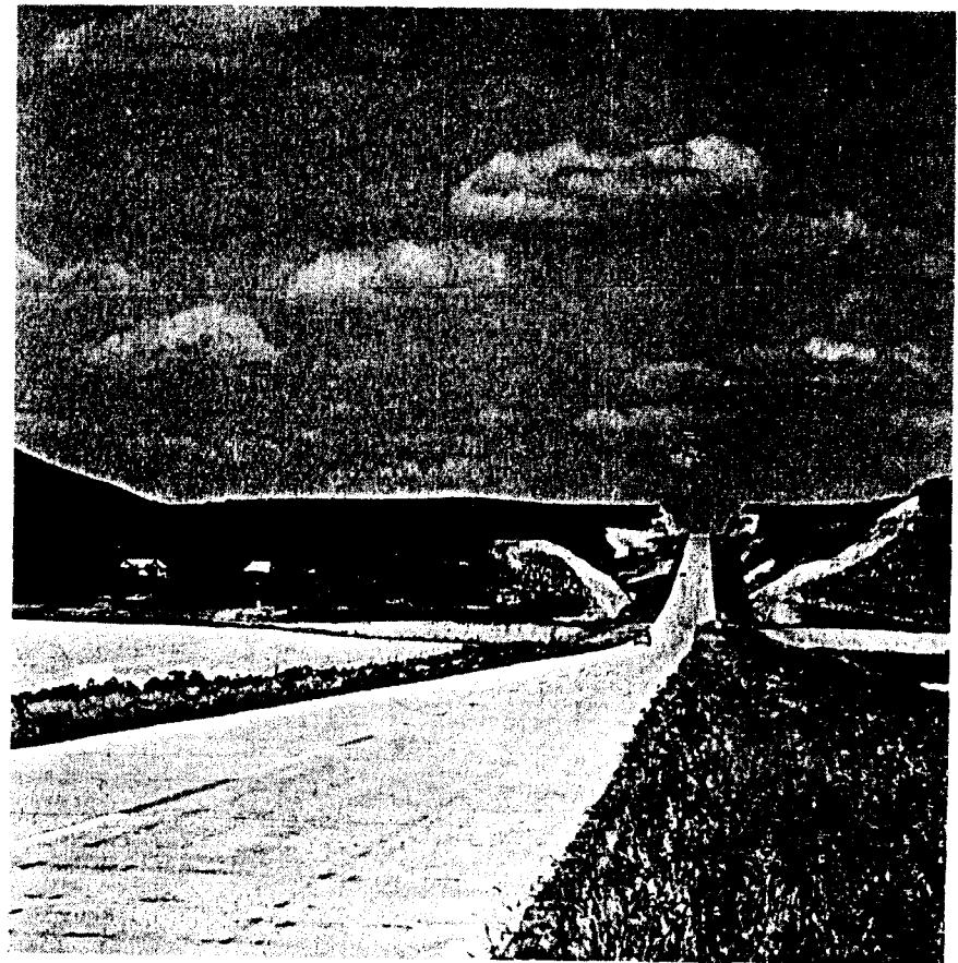
Lack of integration with the landscape. A state highway in Kansas.
