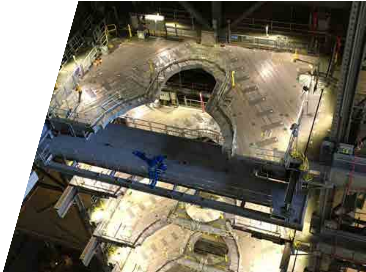
Construction Aid Platform Photo credit: RS&H/Mike Kendrick 32
