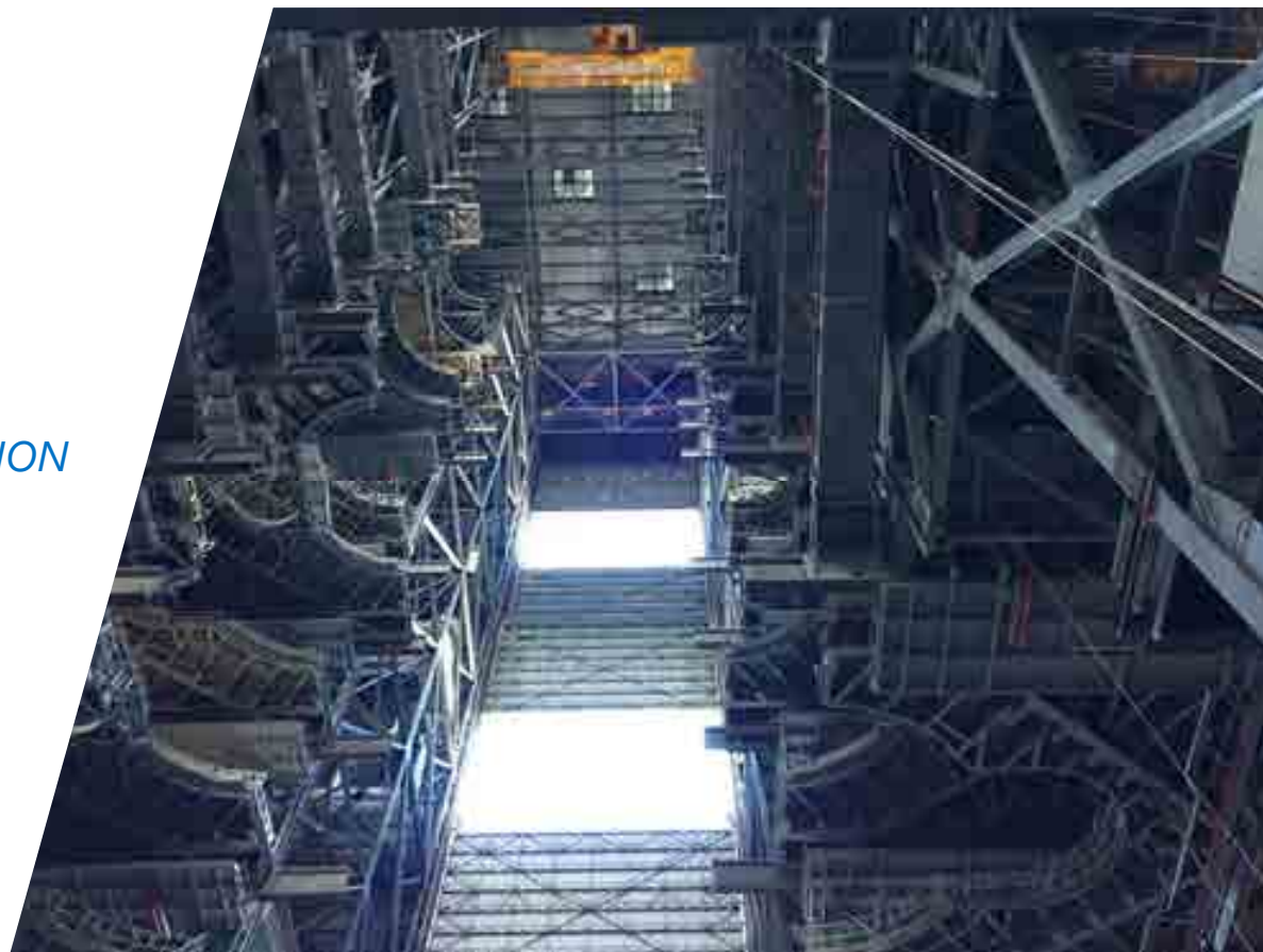
View of HB3 today, looking up to the 325-ton crane. Photo credit: NASA
