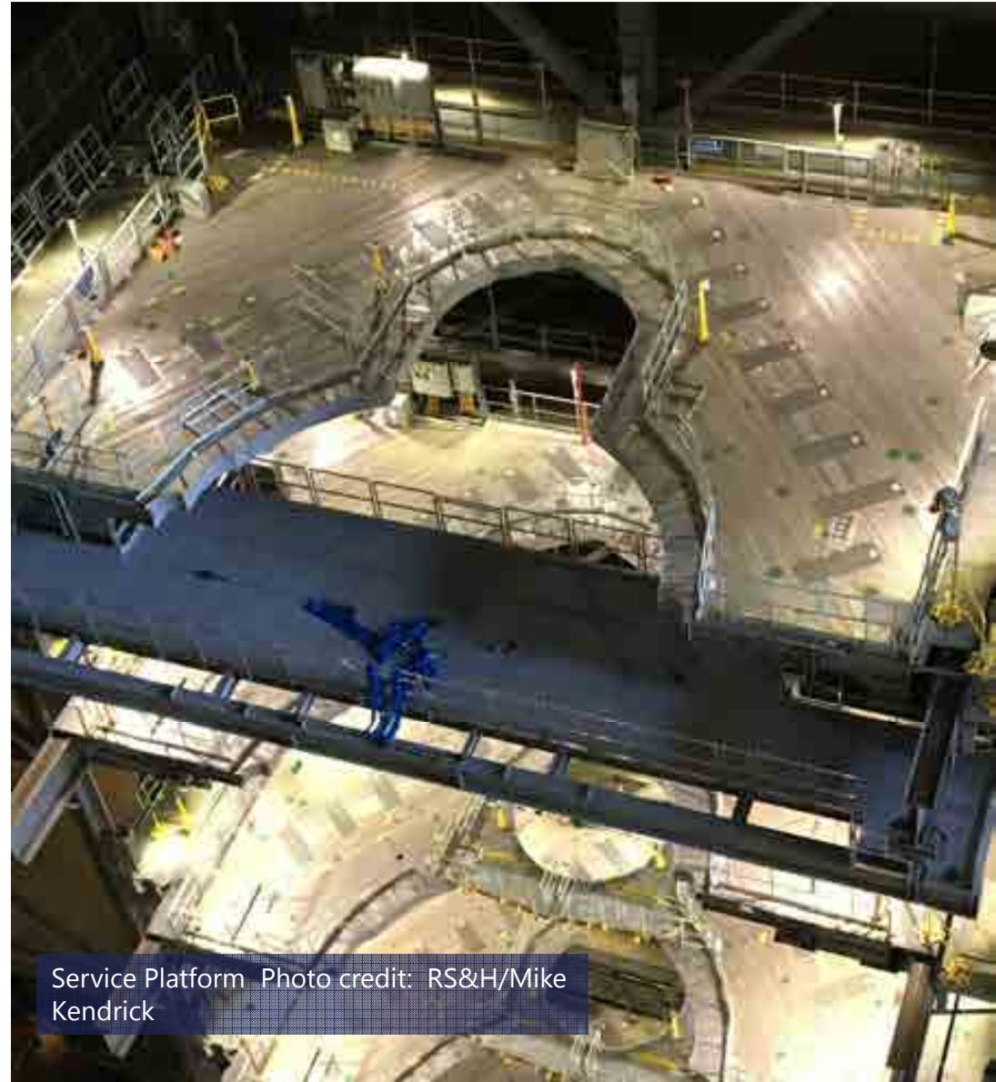
Final Platform Installation Photo credit: NASA/Frank Michaux
