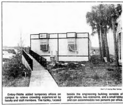
Embry-Riddle added temporary offices on campus to relieve crowding experienced by faculty and staff members. The facility, located beside the engineering building consists of eight offices, two restrooms, and a small lobby and can accommodate two persons per office.
