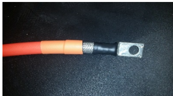
Figure 97: HV Cable step 7
