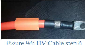
Figure 96: HV Cable step 6
