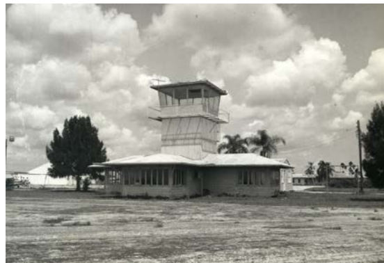
Looking NNW towards the tower
