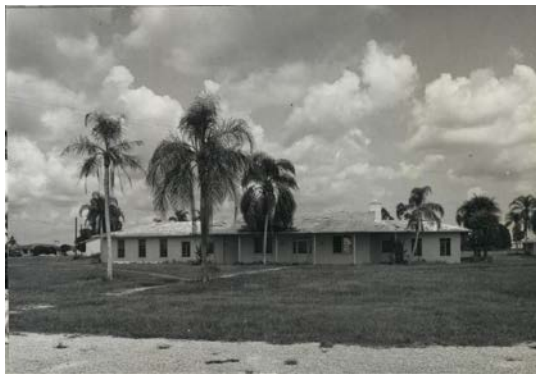
Looking N towards the front of the canteen. The building was still in excellent condition complete with soda fountain although not in use
