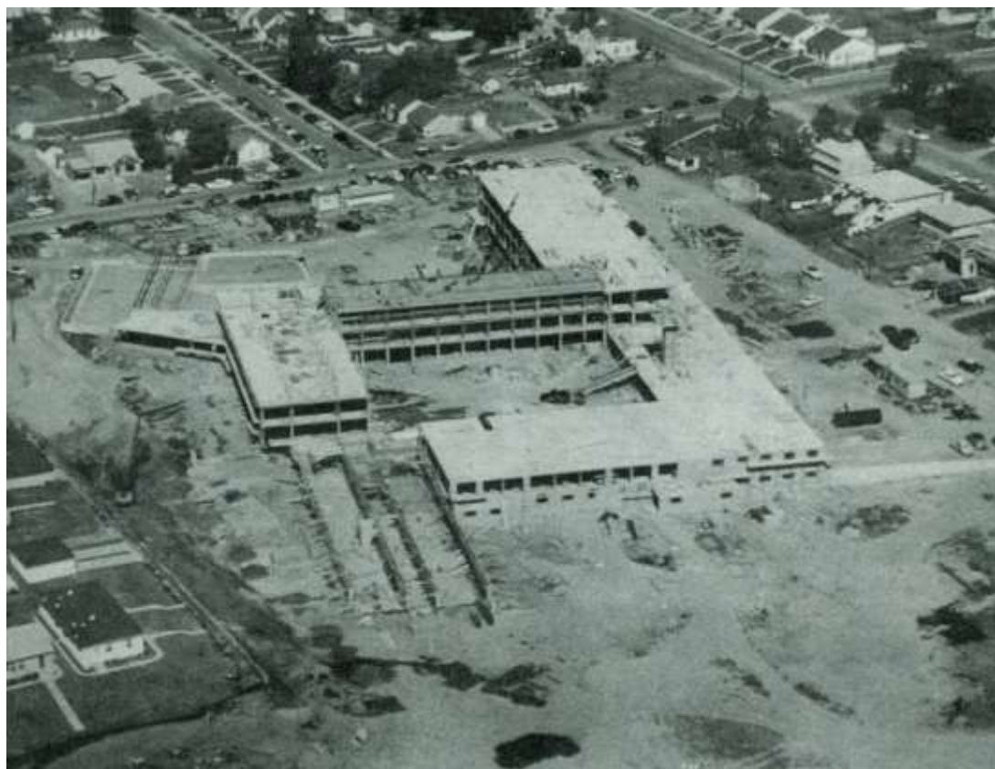
4 - Construction of the New Robbinsdale High School
