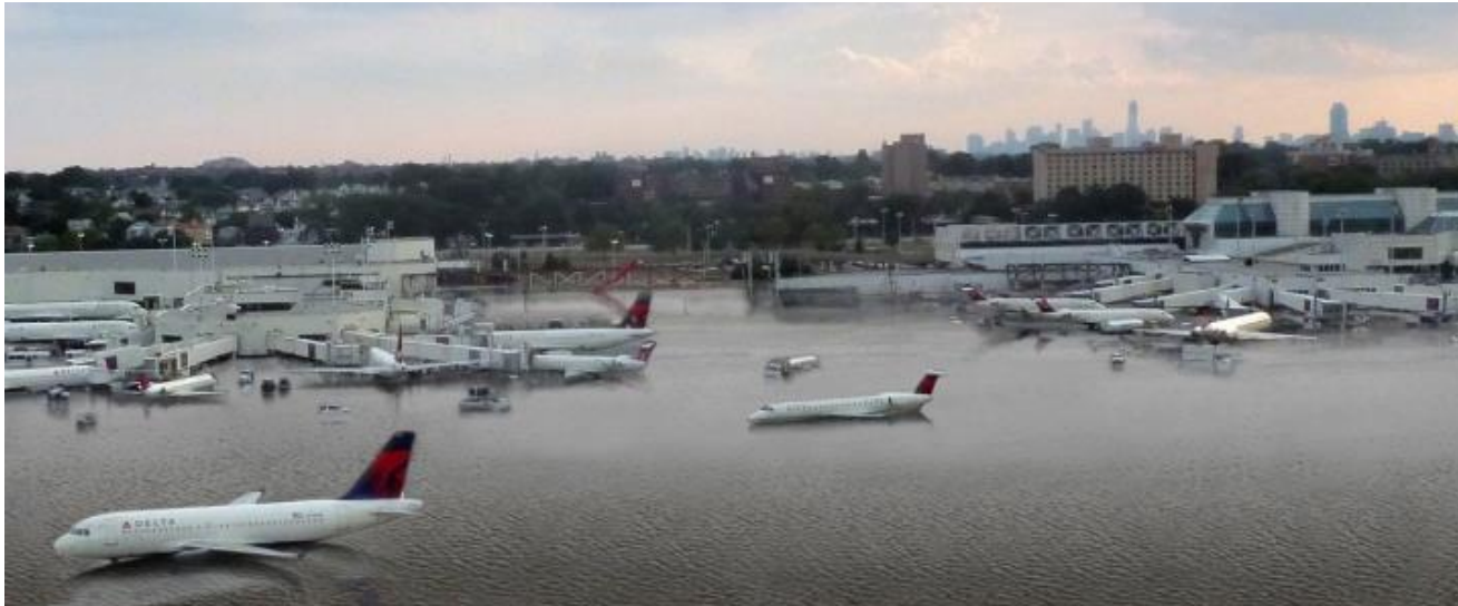
LaGuardia after Hurricane Andrew
