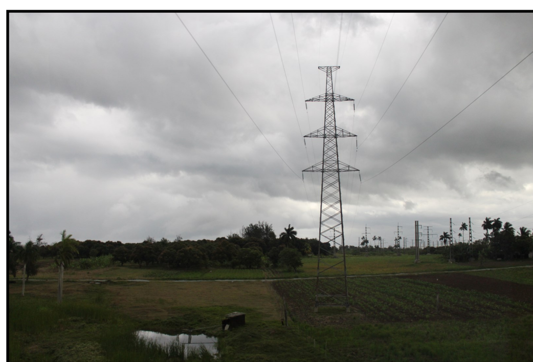
Cuba's electricity grid extends far out into the country. Most, if not all of the energy grid is above ground.
