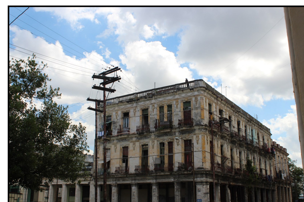
Phone lines cross each other in front of a dilapidated building, providing connectivity to the people.
