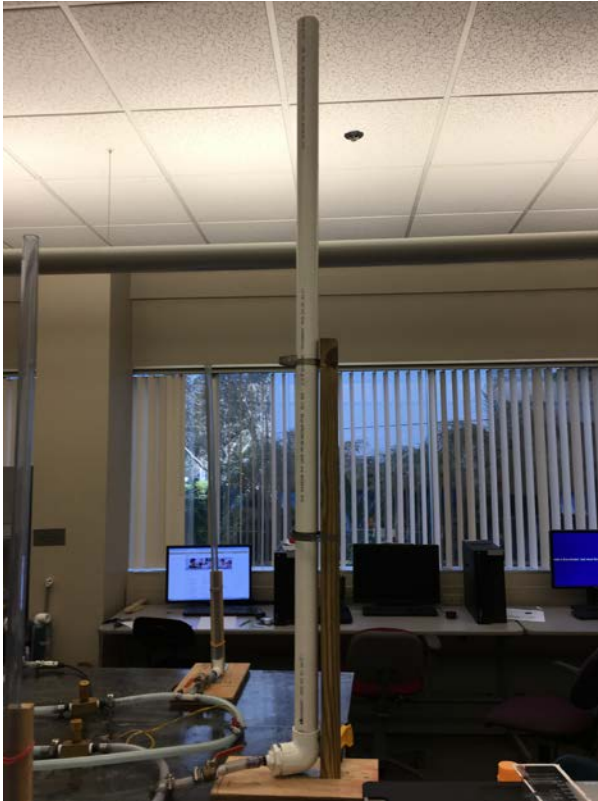
Figure 4.1: Figure showing a compliance chamber installed in the MFL
