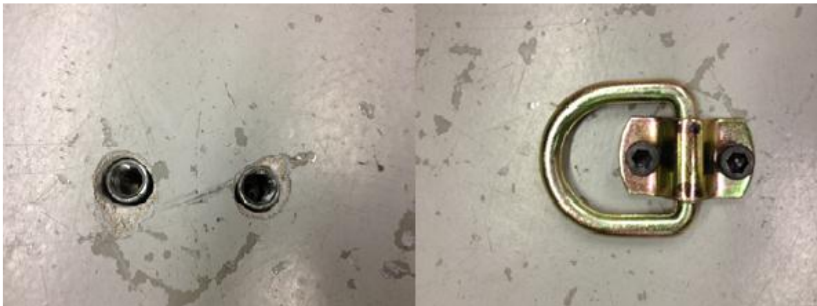
Figure 3.17: Floor Anchor with D Ring
