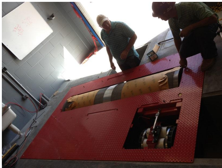
Figure 3.20: Deck Plate Installation
