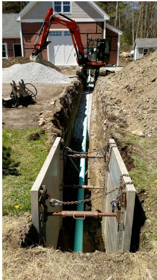
Installation of a house service
