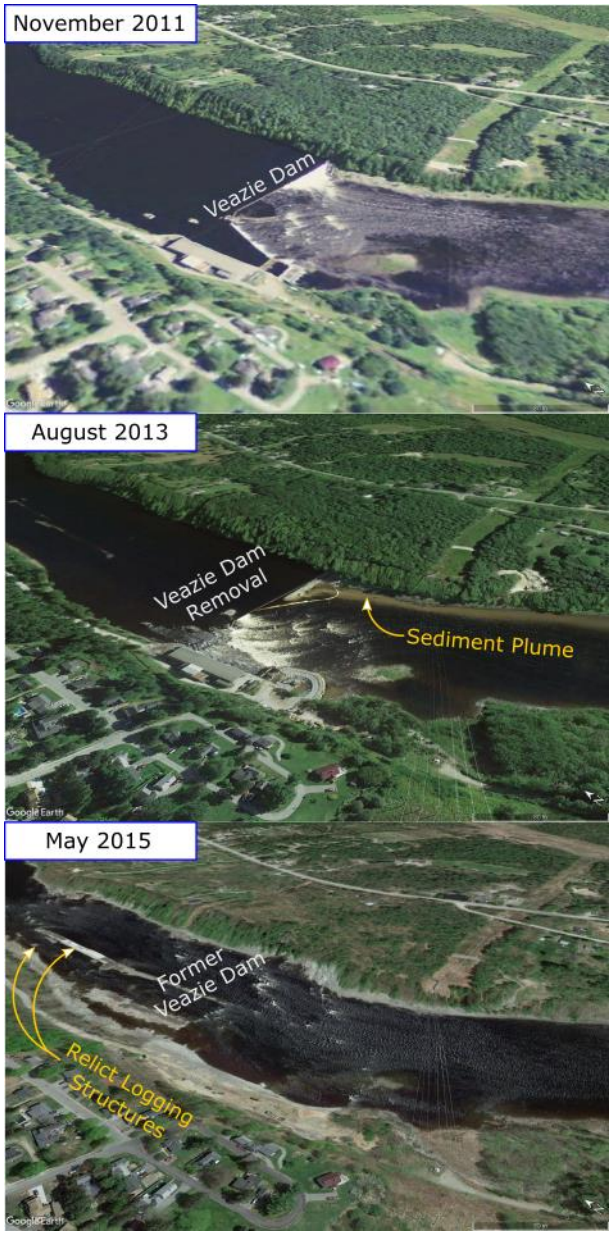
Figure 3.2 – Images of the Veazie Dam Removal: Before, During, and After
