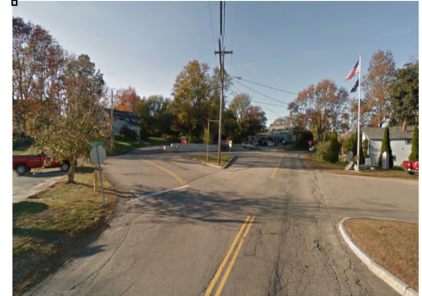
Intersection of State Road and Rogers Road, one of the high crash locations.
