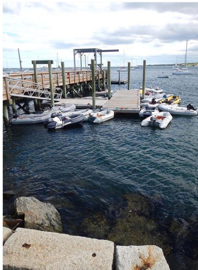
Dinghies tied up at Fishing Pier at Pepperrell Cove, the primary Town-operated mooring facility
