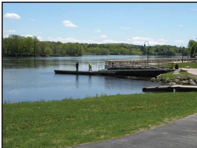
Public Works setting up the docks at the Gardiner Landing
