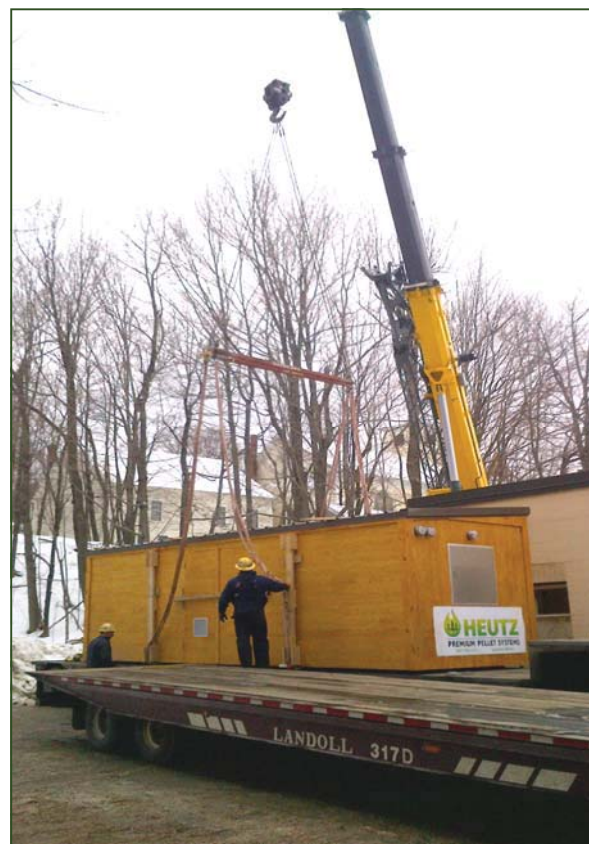
Heutz installing a new pellet boiler at City Hall.
