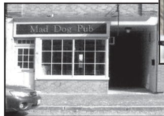
Front facade before...
